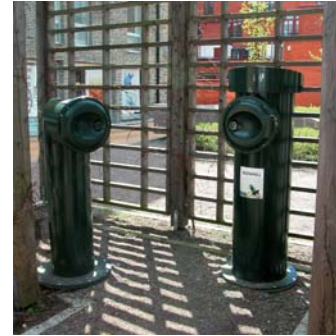
Image 79 Domestic waste chutes to underground storage, Malmö
