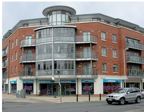
Image 87 Mixed-use building with active frontage
