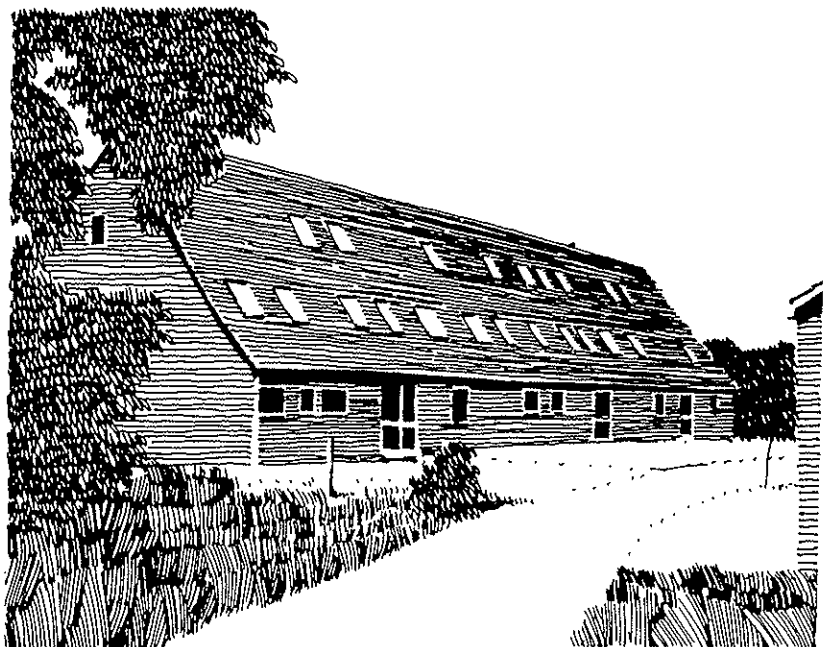
Barn at Hatfield Broad Oak, converted to three houses — entrance side. Architects: S. Peachment and P. Nixon.
