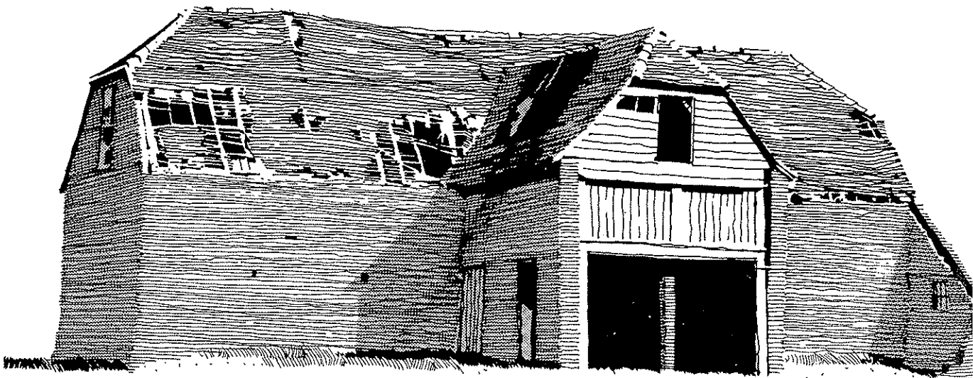
A late brick barn at New Marsh, Foulness, demolished in 1975.
