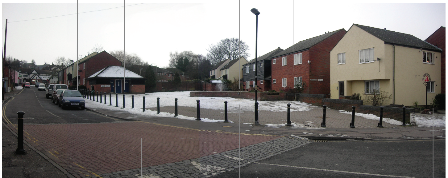
Crossing point fails to pick up pedestrian desire lines across the wide junction
