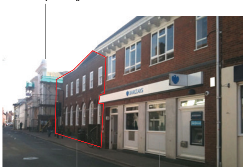
The sorting office is set back from the building line
