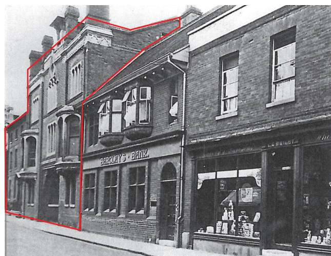
Apart from windows and fixings Barclays remains the same
