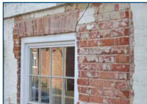
Building currently undergoing paint removal
