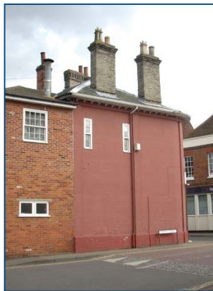
Painted flank wall, Manningtree High Street
