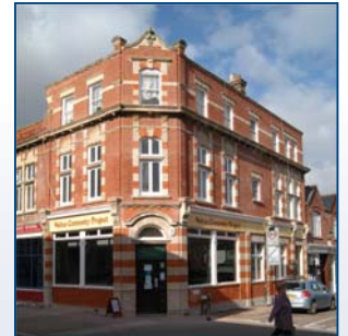
Former Barclays Bank (now Walton Community Project) before and after paint was removed
