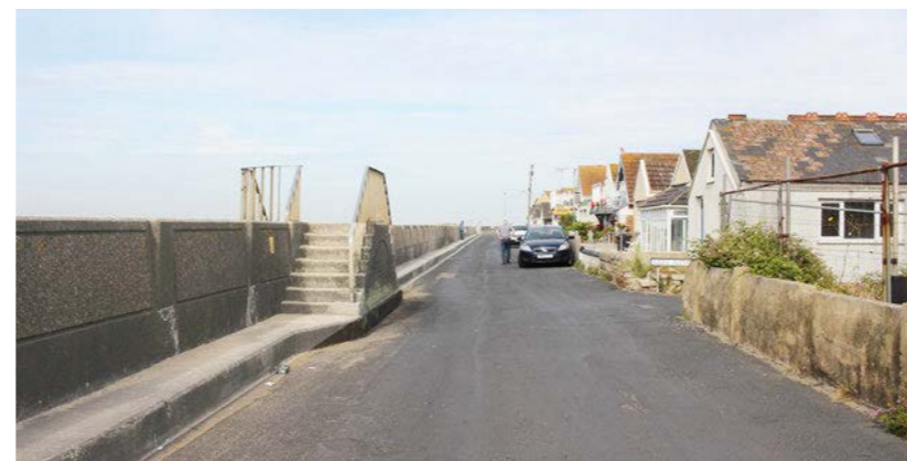
Fig. 75. Photograph of current condition of Brooklands
