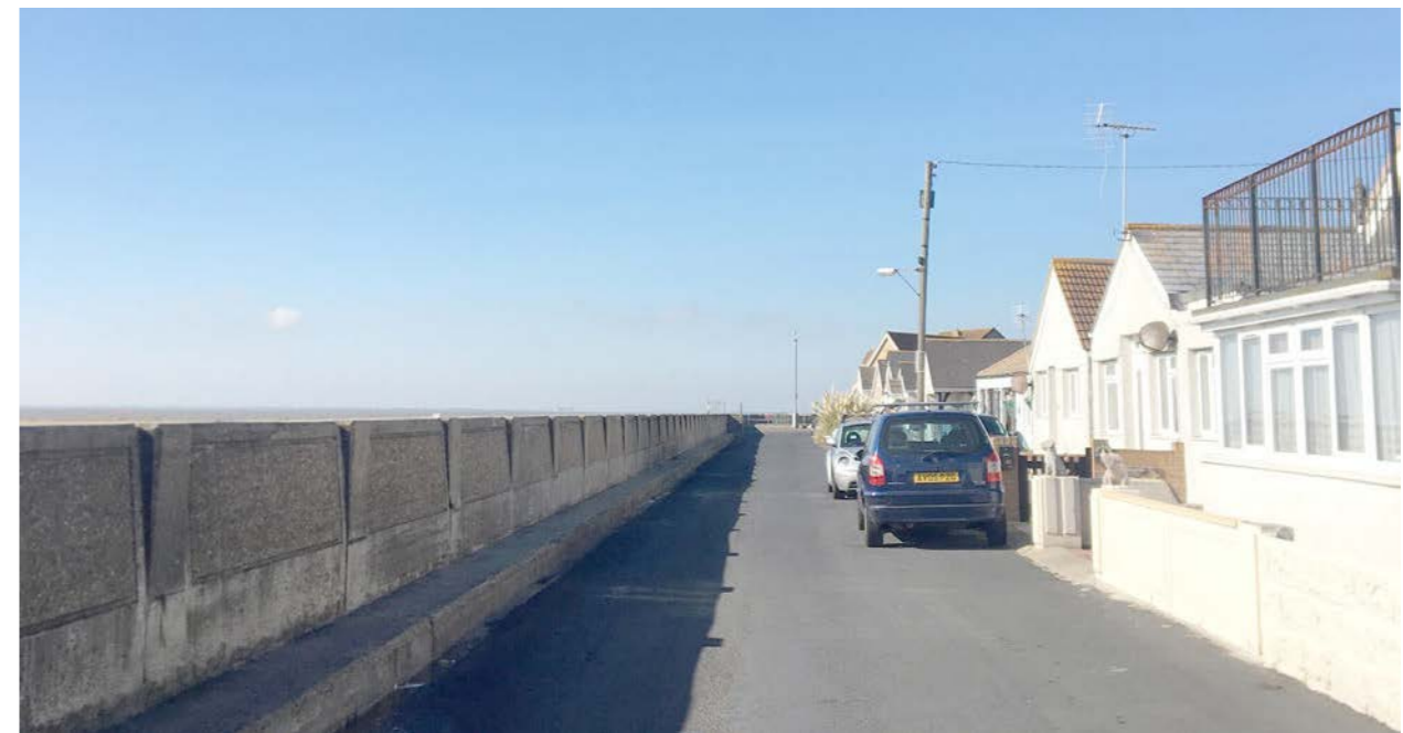
Fig. C33. View of Village seafront (DU3) - current condition
