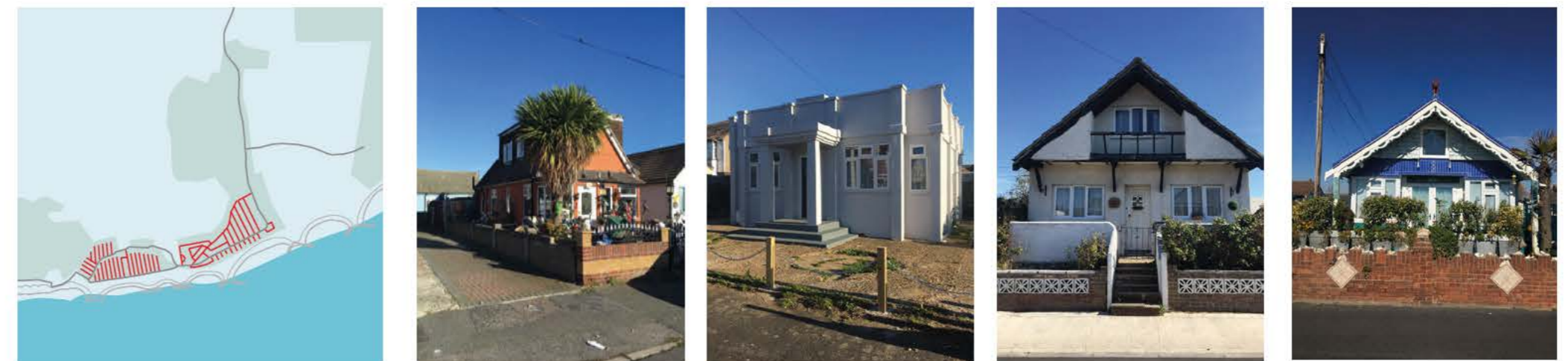
Fig. 57. Map and photographs showing the unique pattern and character of buildings found in Jaywick Sands
