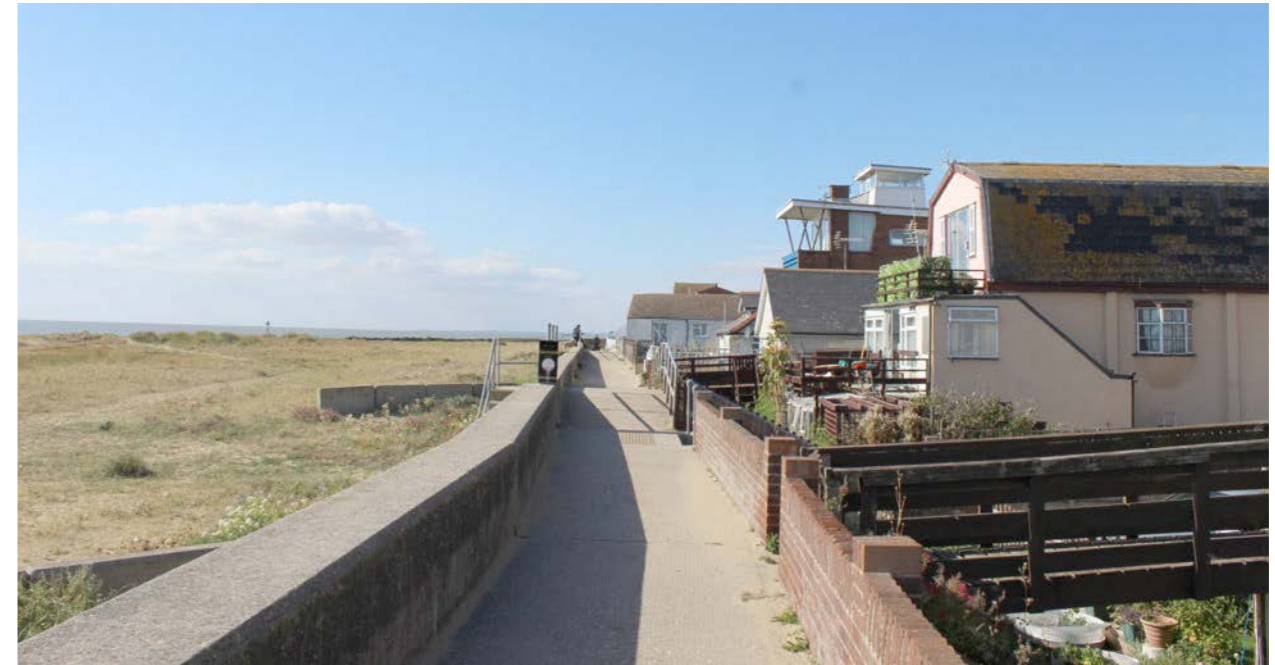
Fig. C18. View of Village seafront (DU3) - current condition
