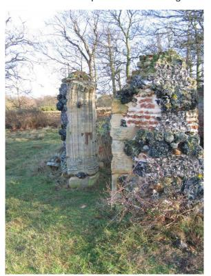
Figure 45: All that remains of the ruin of the Grotto, a folly remarkable for its exaggerated rustication and the reuse of a fine 13th-century doorway.
