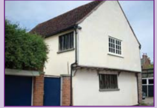
15th Century timber framed and plastered out building, Manningtree
