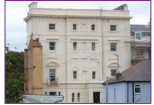
Part of Orwell Terrace, Dovercourt - Roman cement render
