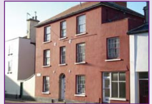
Clear Ashlar effect seen on front elevation of Wellington House
