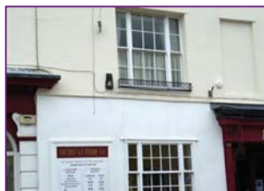
Rendered ground and first floor elevations Listed Buildings in Church Street, Harwich
