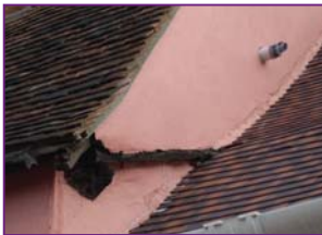
Detail of plasterwork / roof junction
