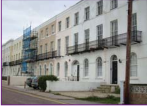
East Terrace, Walton - Stucco frontage
