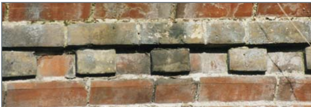
Victorian industrial brickwork detail
