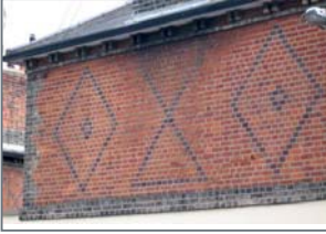
Local example of diaper patterned brickwork
