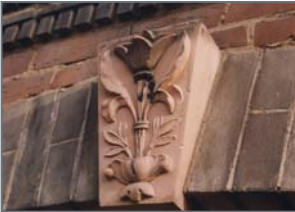
Window arch detail in terracotta
