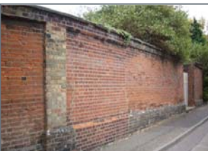
Important boundary wall to Listed Building in Harwich with repaired section
