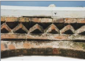
Victorian industrial brickwork detail
