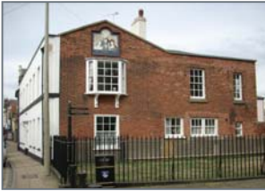
Impressive flank wall of the former Three Cups Inn, Harwich
