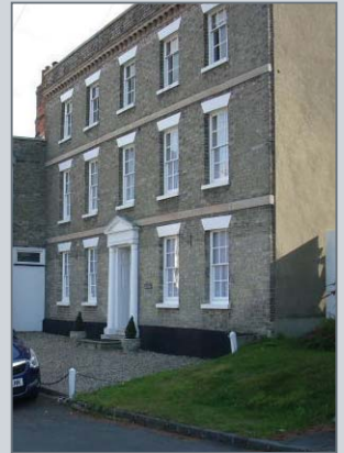
Gault brick facade of Listed Building in Manningtree
