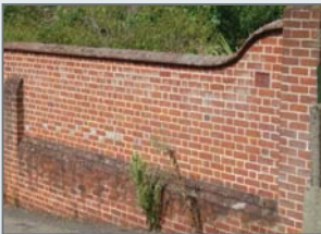
Re-built historic wall (Flemish Bond)
