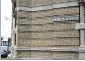
Yellow Gault brick with stone dressing former Great Eastern Hotel, Harwich
