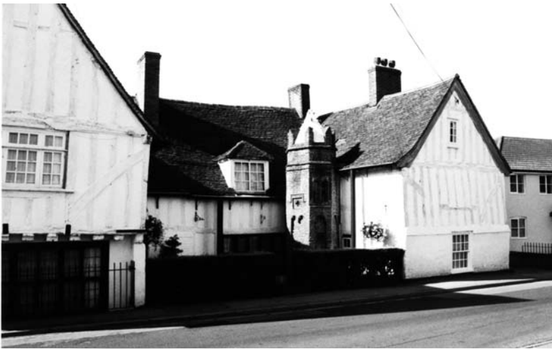
5. Jacobs is an exceptionally fine late medieval house, and is chiefly notable for its Tudor stair tower. The house is, however, only the best of a number of fine medieval properties in this part of Brightlingsea.
