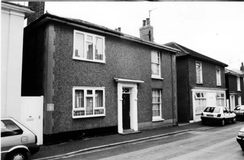
16. Two houses, made grander by positioning one front door on a side return. It is unfortunate that the property with the beautiful door case also has plastic windows in openings of altered proportions.
