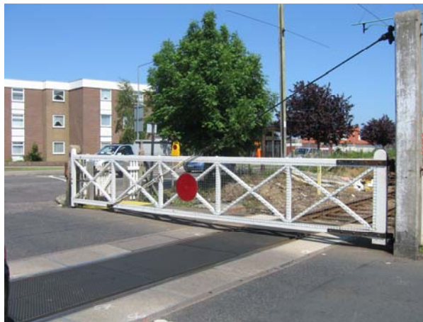
The level crossing gates are both a real and a symbolic entrance to the town. There is much scope here for visual improvements that can be provided through active management.
