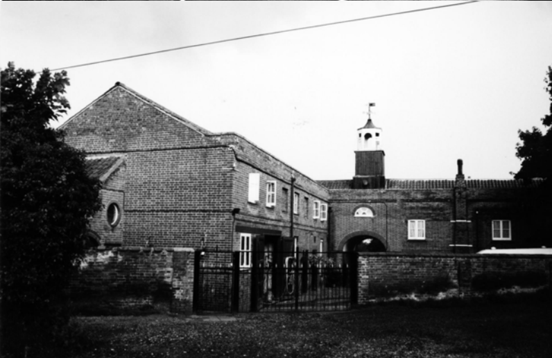
27. Situated close to the confluence of various paths and rights, this survival of the former Mistley Hall is itself something of a focal point. Its brick elevations contain many attractive features, and the boundary wall is a prominent part of the Area.
