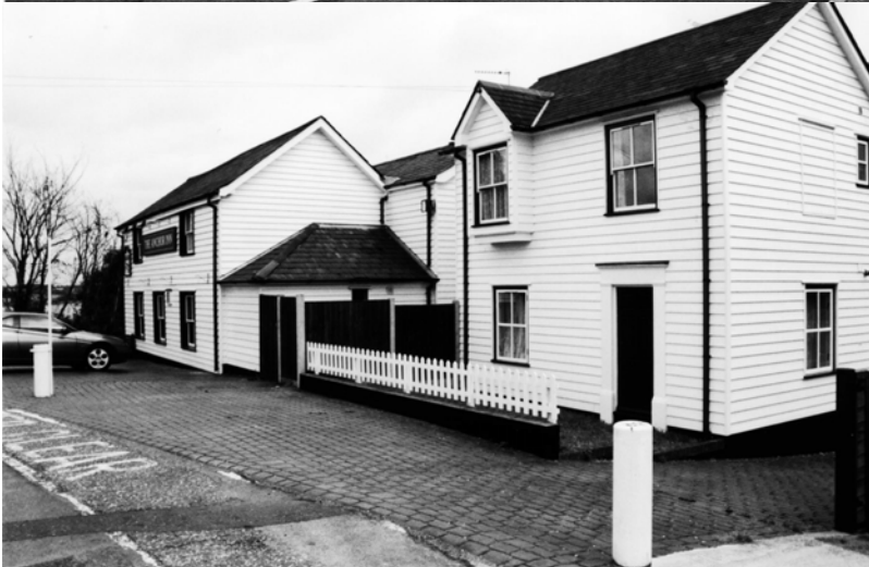
22. The Anchor Inn and the new house next door are maintained under their weatherboarded facades. The loss of the chimneys to the original building is regrettable, and the printed concrete forecourt has an insistent quality not shared by its relative openness to the street.
