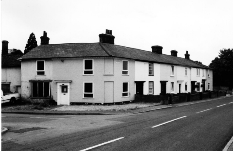
21. James Terrace at the eastern end of High Street is a significant part of the development history of Mistley. Though it retains its slate roof and door cases, the terrace has lost all its original window details, a particular problem given its prominent setting.
