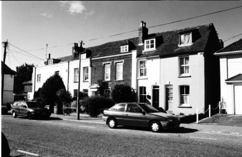
4. These properties east of John Street in the wider part of the High Street show considerable evidence of reworking over the years. Apart from one or two regrettable features, they are an important part of the specific character of this intermediate part of the High Street as it runs into Hurst Green.
