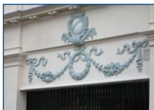
Plasterwork detail from the Electric Palace, Harwich
