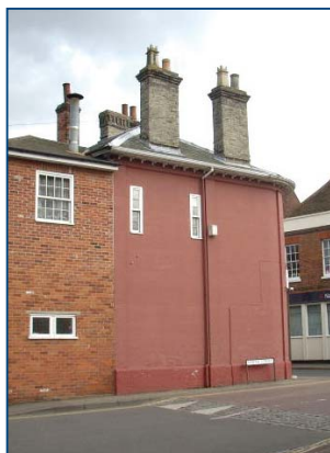
Painted flank wall, Manningtree High Street
