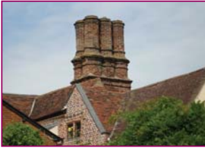
Above: Various chimney stacks in Manningtree
