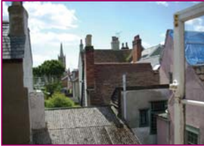
Harwich roofscape looking towards St. Nicholas Church
