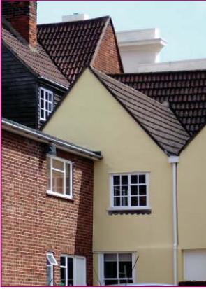
Rear extensions of various forms including inappropriate flat roofed structure
