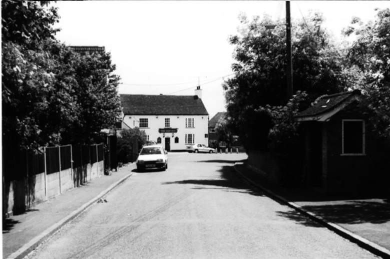
3. The Ship Inn is prominent in views towards the square and is its major defining building. Walls and trees help to define the view: the brick wall on the right is more sympathetic than the concrete blockwork on the left.
