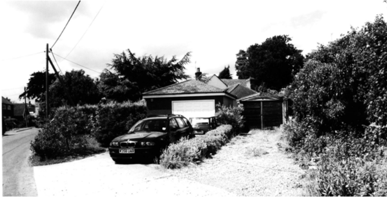
10. Accommodating the private car requires considerable thought and ingenuity to find satisfactory solutions that retain the character and appearance of private land in historic settings. While these drives and garages are no doubt useful, their location, design and details do not enhance the rural character of Church Lane.
