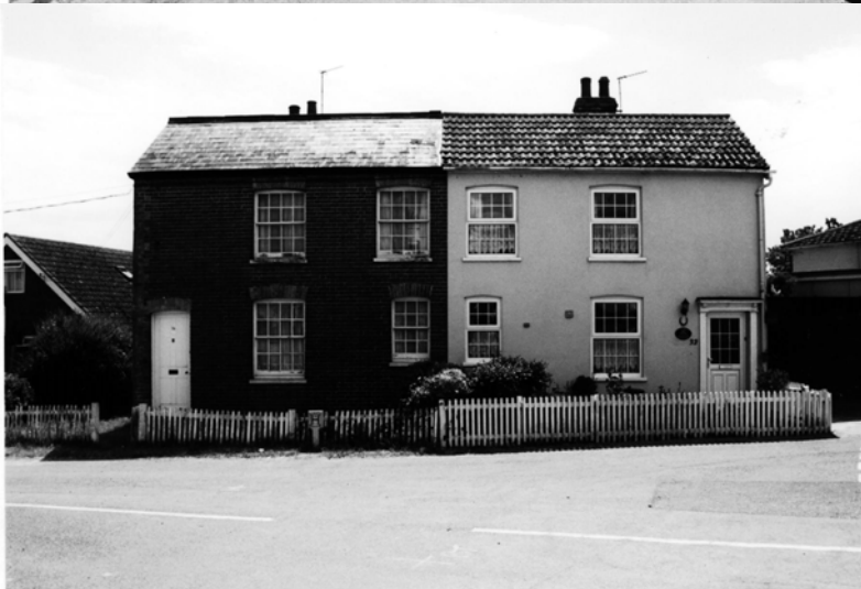
4. Nos 32 Ash Cottage (right) and 34. This modest pair of cottages gains additional importance from their formal relationship with other buildings in the square. The survival of original facing materials and joinery at no 34 demonstrates how much original character has been lost in the Area in the last fifty years or so.
