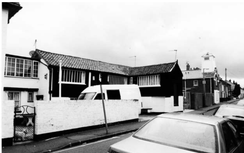
17. The rear yard of The Galleon forms an attractive group with the Board of Trade wreck warehouse at the foot of Sydney Street. The pantiled roof is an attractive feature, and always looks well with weatherboarding.
