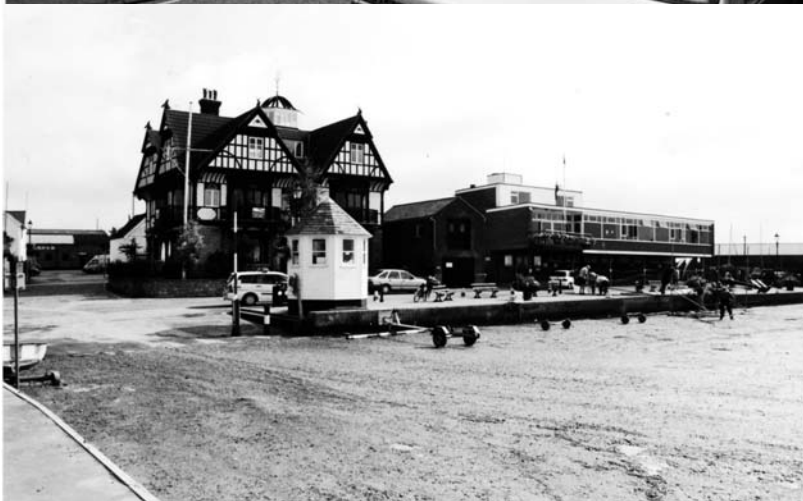
18. There is a strong contrast between the Jacobean styling of the former Anchor Hotel, and the nautically workmanlike façade of the Colne Yacht Club. Conversely, the flat-roofed character of the Boat Centre on Waterside is not appropriate given its street setting.
