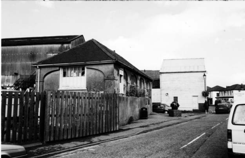
19. The Wreck House is an important survival, though its small forecourt could do with some visual improvement. Together with the adjacent boathouses it forms an important part of the enclosure of Waterside independent of the James and Stone yard to the south.
