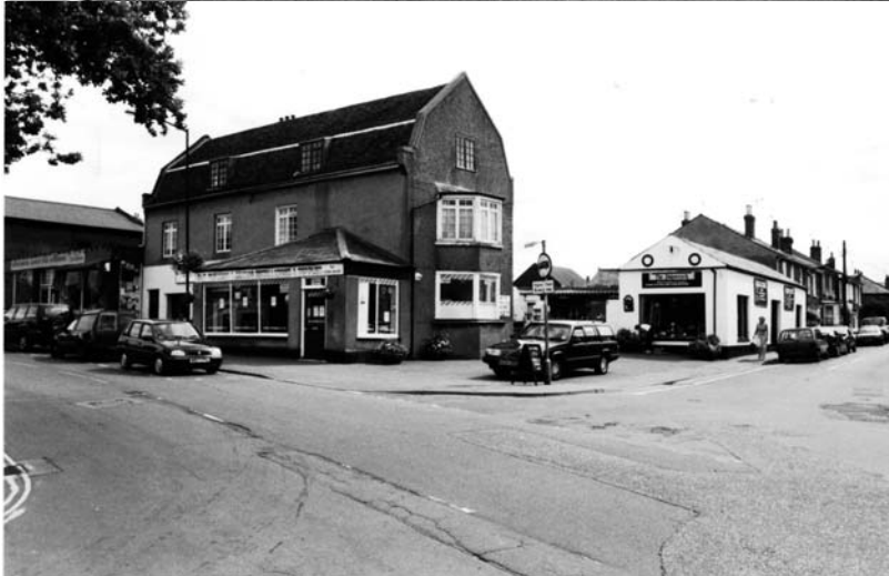
11. This building is prominent in views of Lower Green Gardens, particularly from Station Road. It is much altered, and is somewhat detached from its neighbours by its open frontages. The extent of patched tarmac in this view is also of significance.
