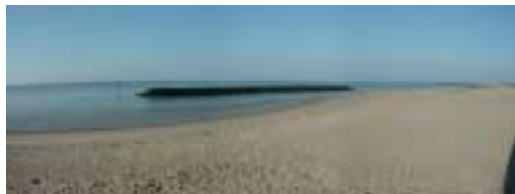
An example of an offshore breakwater holding in place a sand beach
